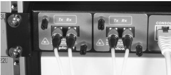
Remove fiber cables
